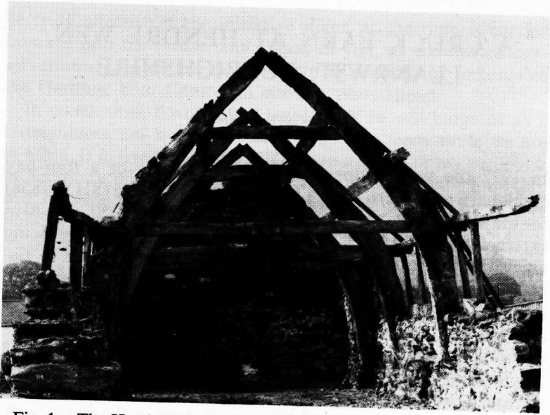
Fig. 1. The Hendre Wen barn before removal: view from the south
